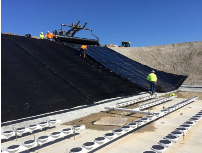
New Basin Liner being Installed – SWWTP
