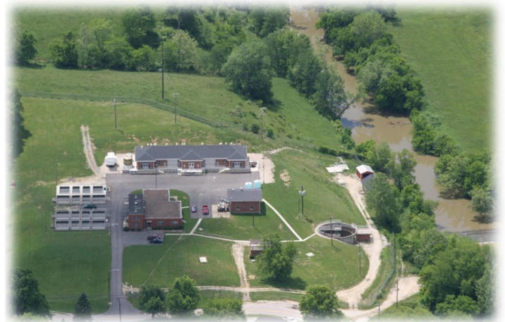
Aerial View of Mt. Sterling Water & Sewer Water Plant
