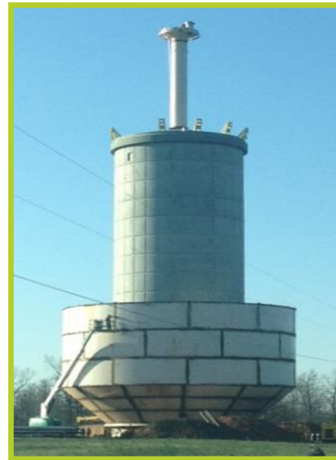
The Springfield one-million gallon tank under construction.
