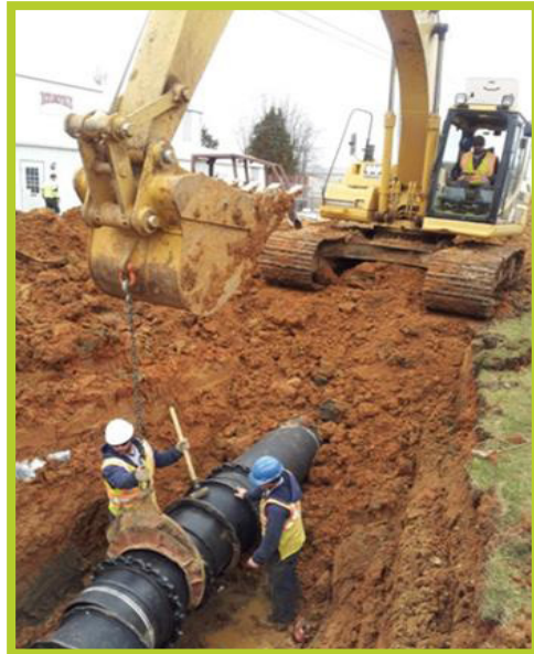
Pictured is the last piece of 24" pipe being installed.
