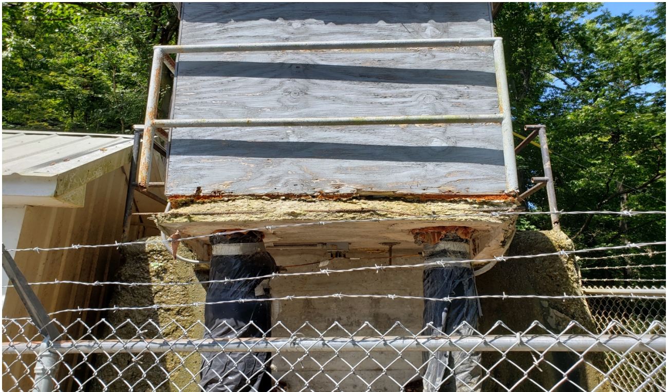
Raw Water Pump
