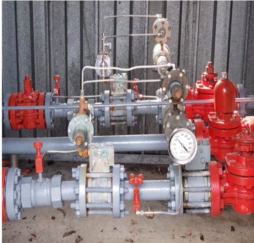
Logansport Main Regulator Station.
